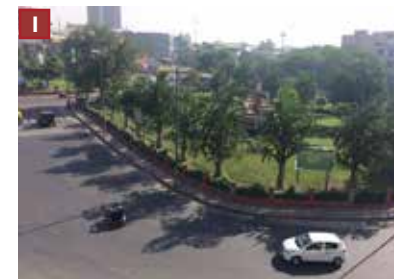
Pusa Roundabout It is a 5 arm signalised roundabout and is located at the intersection of Patel road, Pusa road and Shankar road which causes a situation of chaos and congestion on the road. Source: DUAC, 2017 [Photograph], New Delhi
