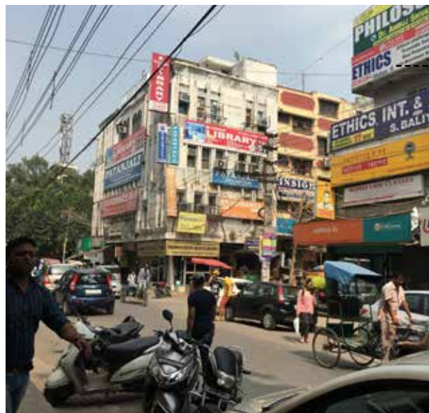
Signage by various establishments disfigure the facade and deteriorate the character of the road.
