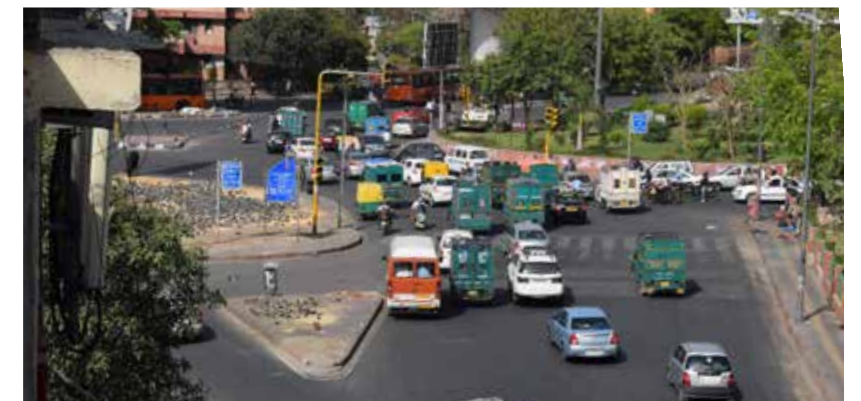
Numerous Traffic islands gives the vehicle more manoeuvrable space which leads into a traffic jam.
