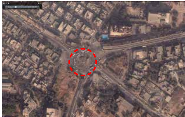
Time Line year: 2004 The size of the roundabout was reduced to incorporate metro piers and also to accommodate the increased traffic volume.
