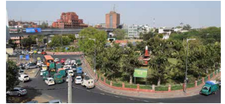
Multiple alternatives for traffic flow (due to numerous traffic islands) leads to gridlock situation
